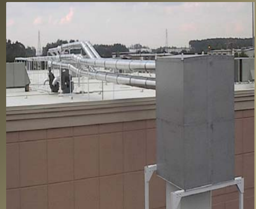
Roof mounted material conveying system
