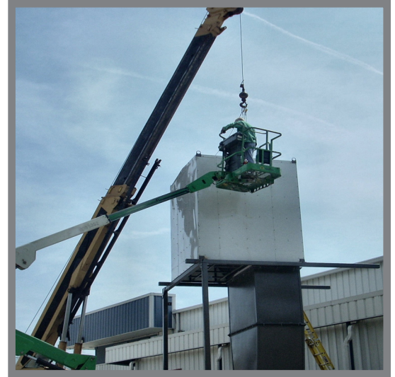
Installation of a weather covered separator
